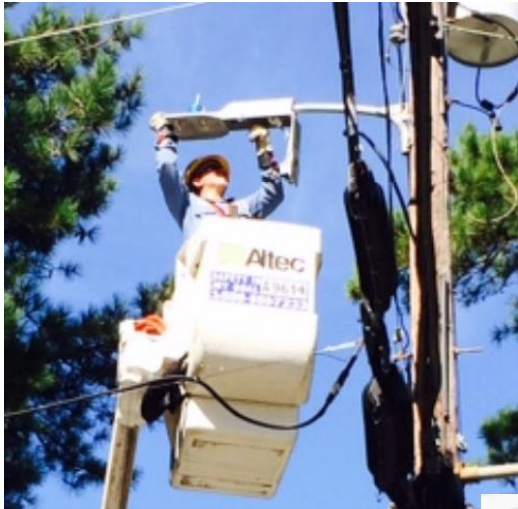
Hinged, Removable Power Door Driver is mounted to door. Integral hinge allows door to hang securely while making wire connections and can be easily removed without the use of tools.
